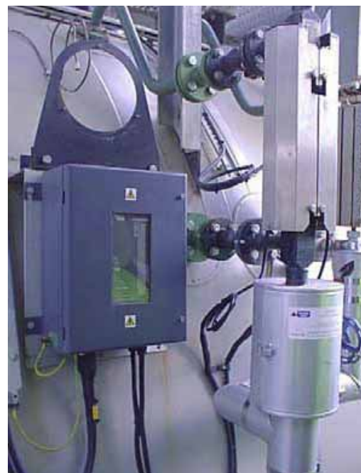
Figure 1: Hydrastep installation
