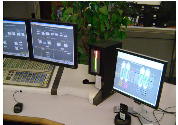
Mobrey Hydrastep remote display, separate to the DCS
